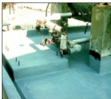
CHEMICAL STORAGE AREAS
