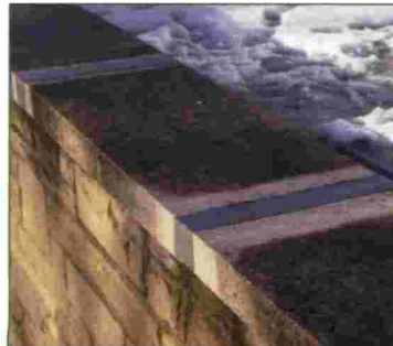
PARAPET WALLS & COPING STONE JOINTS
